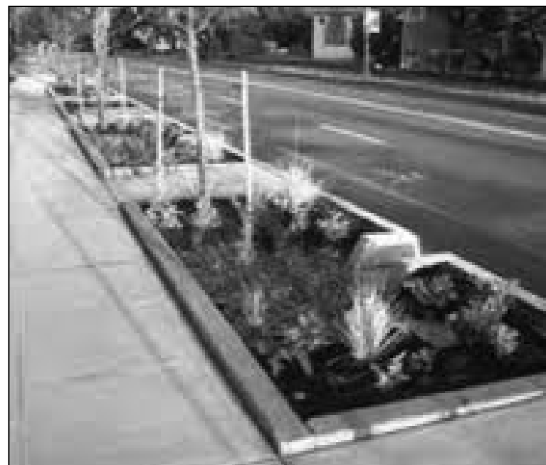
Photo: Courtesy of Portland Bureau of Environmental Services Biovales, such as these in Portland, Oregon, are one way of managing storm water in an urban neighbourhood.
