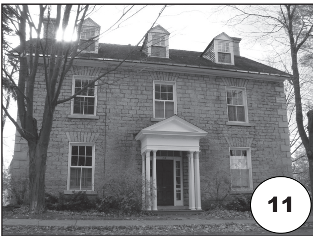
#11. 35 MacKay Street (1864) Allen House. This impressive 2½ storey house on a corner lot at Thomas Street has two entrances and two fine facades of dressed stone (compare with the rougher stone at the rear and side). It was built to accommodate senior employees of Thomas McKay's mills. Note also the strong cornerstones ("quoins") and fancy wooden trim. The porches and pillars were added in the 1920s.
