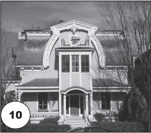
#10. 34 Alexander (c.1864) Henderson House. This spectacular 2½ storey clapboard house is typical of the Second Empire Style and is an example of the evolving architecture of the village. The mansard roof, wishbone-shaped gables, upstairs enclosed sunporch, elaborate wood detailing, impressive front entrance and veranda all blend into an eclectic building of distinctive architectural value. It was built for John Henderson, manager of the MacLaren Lumber Mills. He became Treasurer of the Village of New Edinburgh when it was incorporated in 1866, and later became Clerk of the City of Ottawa.
