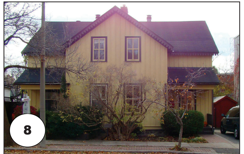
#8. 25-29 Crichton Street (c.1867) McLatchie House. This is the only example of an original "board and batten" double residence remaining in New Edinburgh. The 1 1/2 storey T-shaped structure with its fancy gables was built by W.R. McLatchie as workers' housing in the early years of the village. It has survived virtually unaltered and is beautifully preserved.
