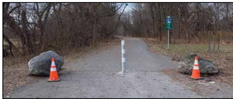
New vehicle barrier installed on the bike path into Stanley Park.
