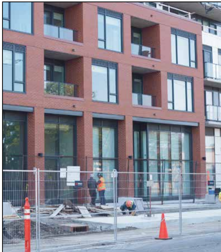
88 Beechwood – A work in progress!
