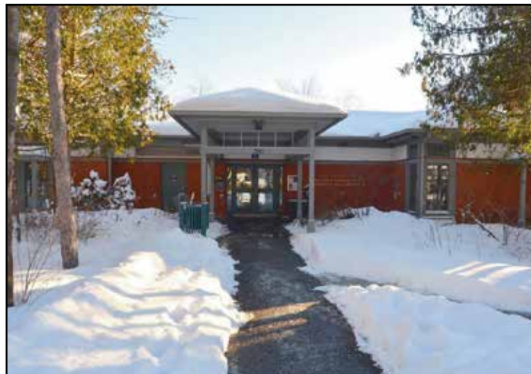
The Rockcliffe Park library branch, 380 Springfield Rd.
